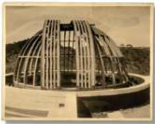
Mountain Boulevard Construction
